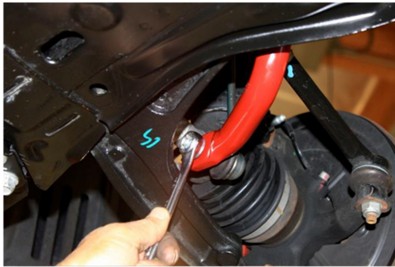
17. Re-install end-link nut using 16mm wrench and torque to 54Nm (40 ft. lbs).
